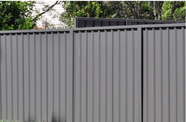
SIDE BOUNDARY FENCE: TYPE B COLORBOND 1.8mm HIGH
